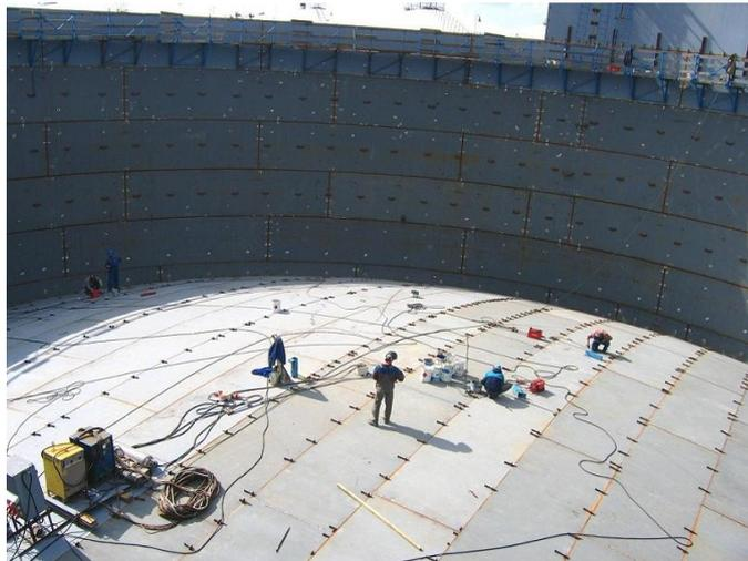
Erection of AST with floating of dome roof
