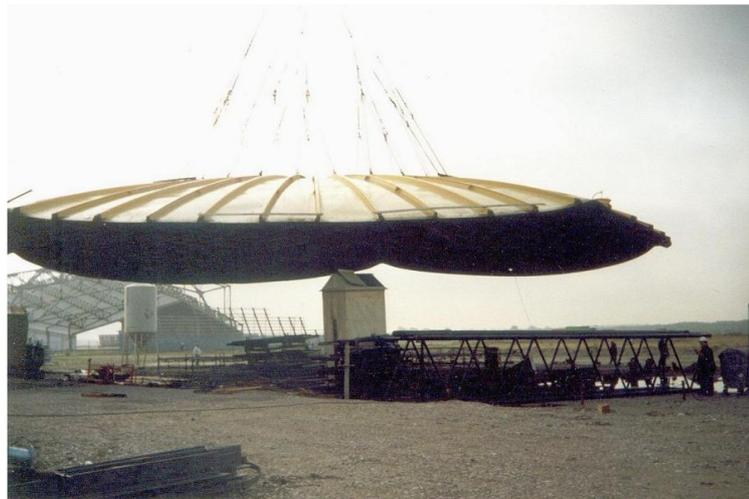
Mounting of dome roof on the shell as one assembly
