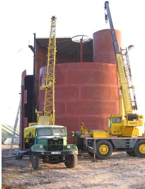
Erection of AST with rolls method
