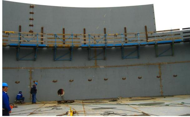
Erection of AST sheet by sheet
