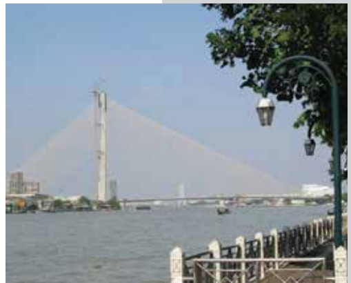
The Rama VIII Cable Stay Bridge - Bangkok, Thailand
