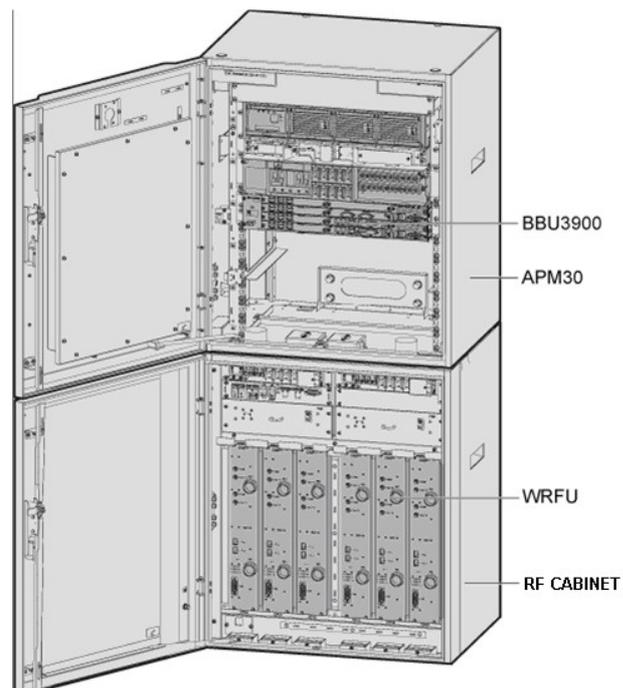
The DC BTS3900A consists of the RF cabinet and the transmission cabinet. The BBU3900 is installed in the transmission cabinet, and the WRFU is installed in the RF cabinet.
